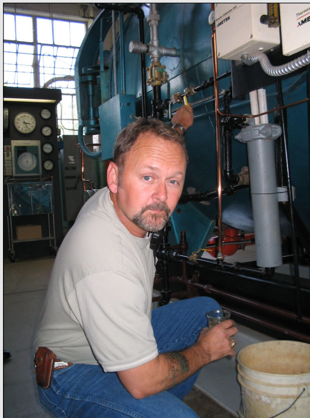
Keith Holt monitors boiler condensate return daily.
