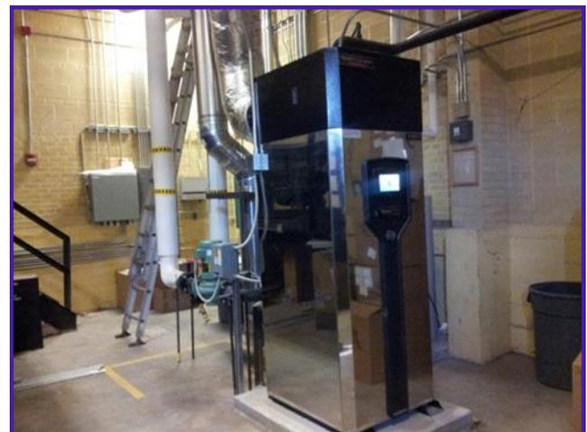
*This low-NO<sub>x</sub>, high-efficiency condensing boiler was installed in 2013. Despite a 20% increase in facility square footage, the new unit used 16% less energy and saved \$1,786 the first year it was operated.*
