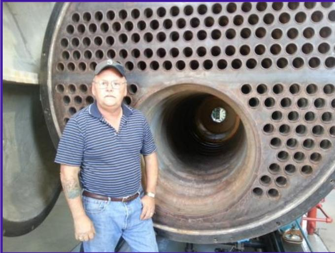
VAMC boiler plant manager, Keith Holt, next to a firetube boiler. Annual cleaning improves heat transfer.
