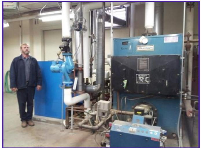
*Lyon County facility manager, Mark McKenna, stands next to the new condensing hot water boiler. The old, less-efficient boiler is on the right and takes up about twice as much floor space as the new unit.*
