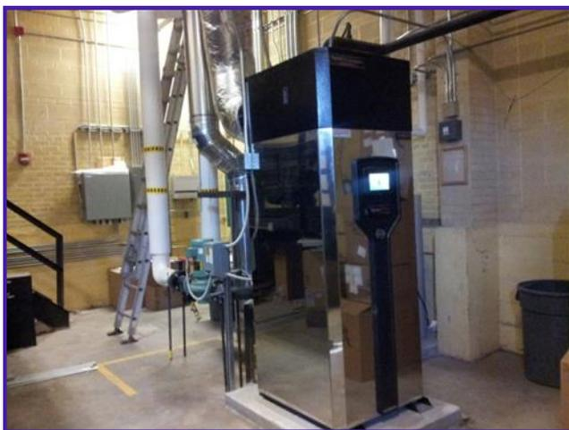
*This Wichita Public School low-NO<sub>x</sub>, high-efficiency condensing boiler was installed in 2013. Despite a 20% increase in facility square footage, the new unit used 16% less energy and saved \$1,786 the first year it was operated.*
