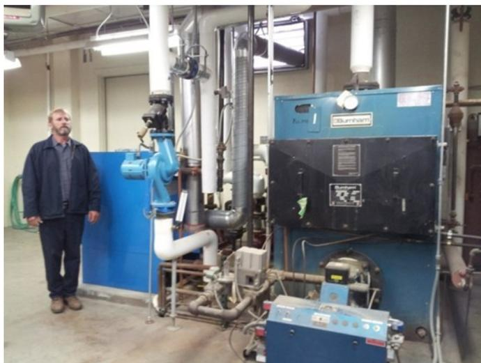
Facility manager, Mark McKenna stands next to the new condensing hot water boiler. The old, less-efficient boiler is on the right and takes up about two-times as much floor space as the new unit.
