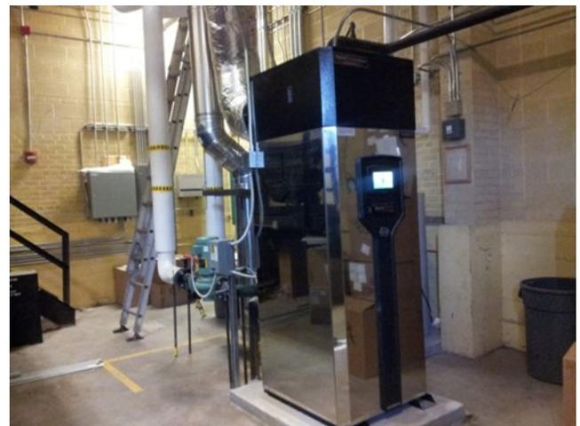
*This low-NO<sub>x</sub>, high-efficiency condensing boiler was installed in 2013. Despite a 20% increase in facility square footage, the new unit used 16% less energy and*
