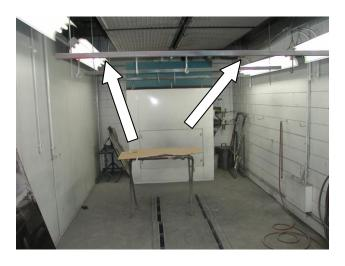
**A.** Yes, a full roof and walls extending to the roof would have to be installed or the spray area otherwise enclosed to meet the full enclosure requirements of the NESHAP.
