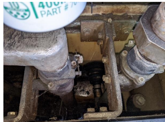
Shear valve anchored with steel bracket
