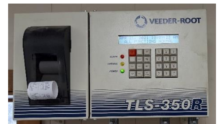
Automatic Tank Gauge (ATG)
