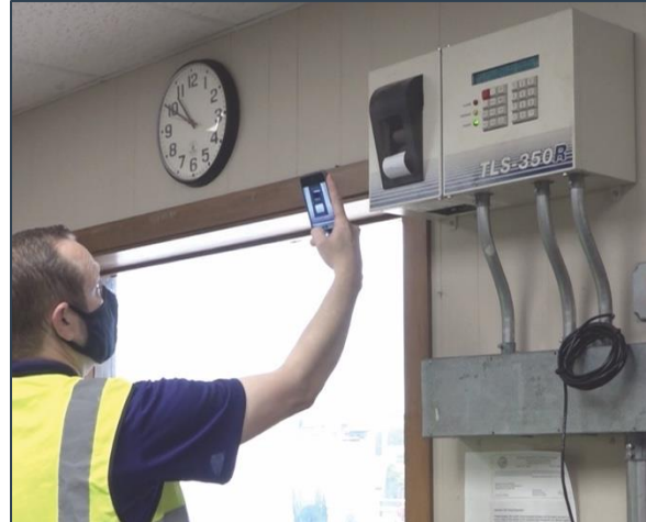
Scanning printouts from your ATG or taking pictures of them will help you maintain records, as the paper used in ATGs degrades easily.
