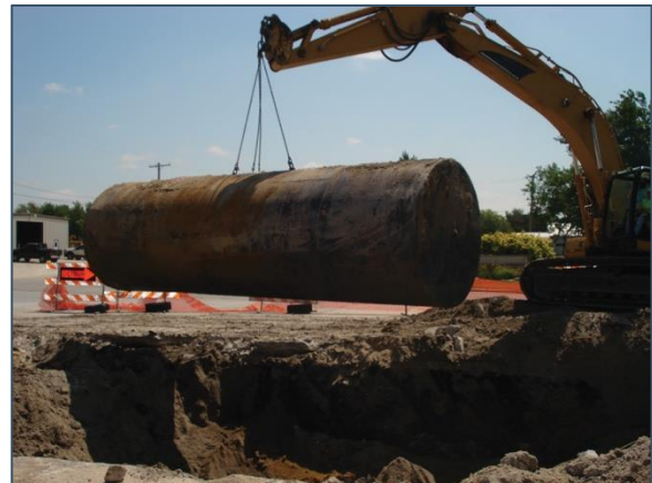
UST being removed from service
