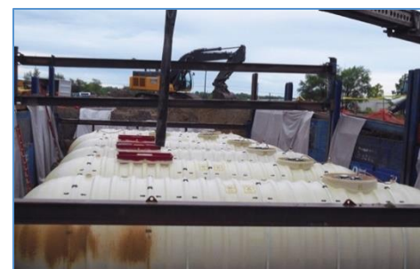
Tank installation excavation showing shoring and bracing
