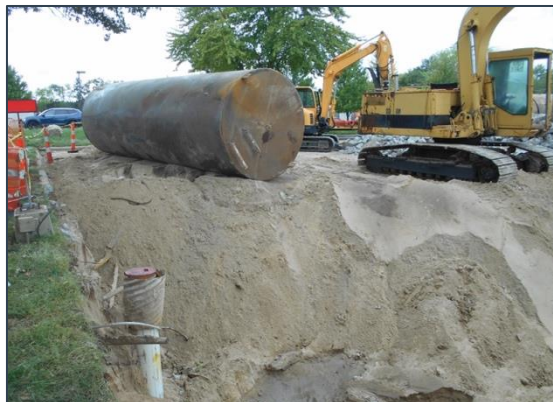
Removal of a tank with evidence of external corrosion
