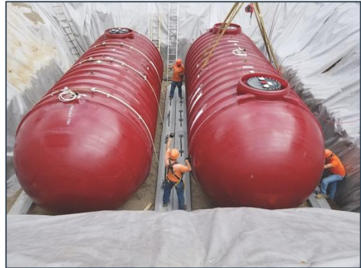
Two USTs mid-installation
