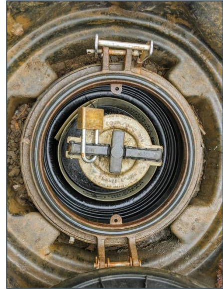
Example of a spill bucket with label inside
