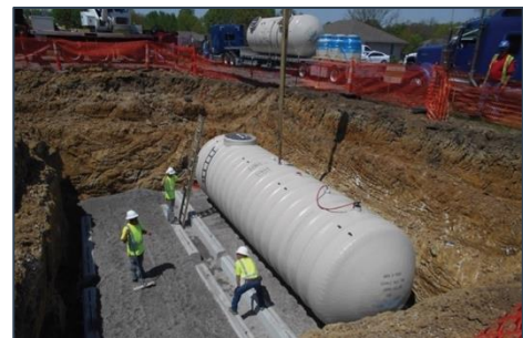
First of two tanks being secured to concrete deadman during installation
