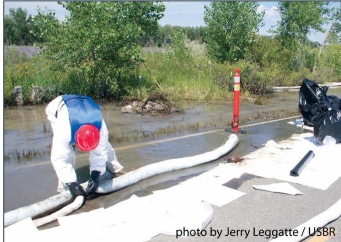
Example of initial abatement: use of booms and spill pads to contain a spill
