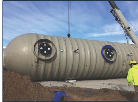
New UST being lowered into a basin during installation
